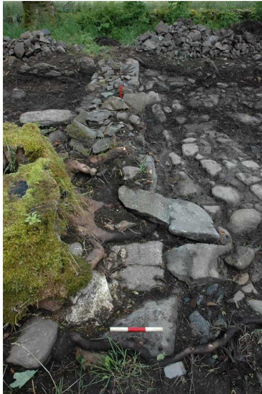
North wall of Building 5 with mortar bonding left of scale
