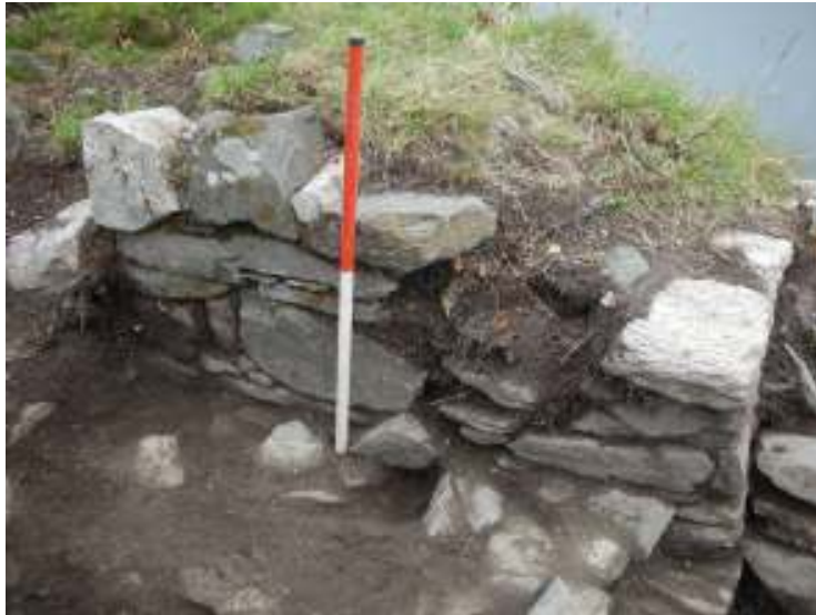
E side of upper enclosure entrance
