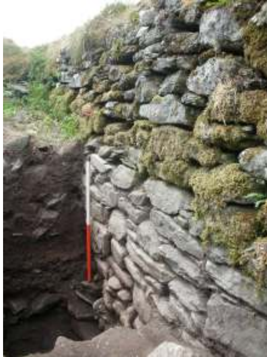
Inner face of upper enclosure [041]
