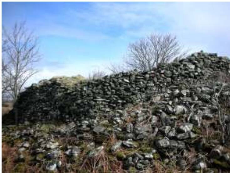
South wall of upper enclosure
