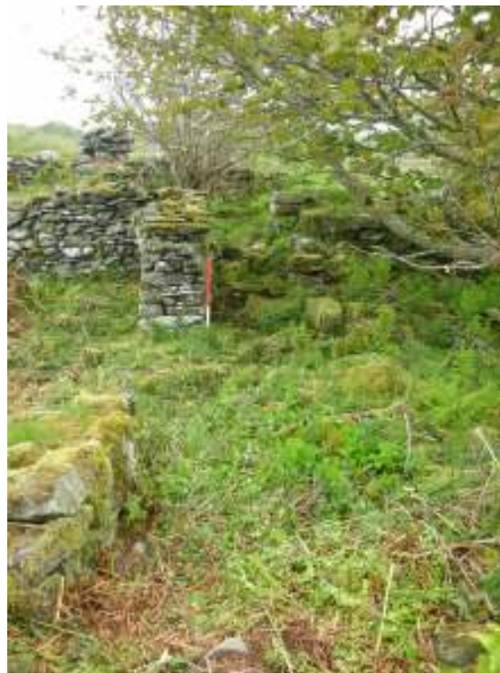
Passage between Structures 1 and 2
