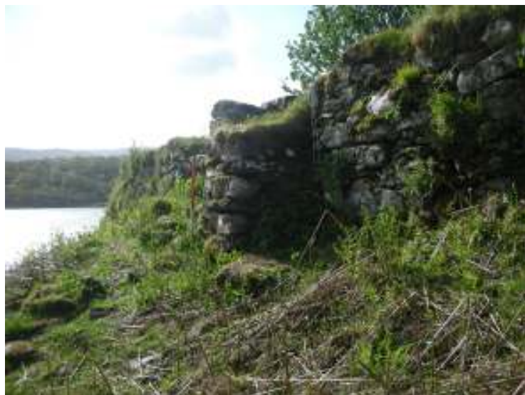
Lower enclosure entrance buttress or pier
