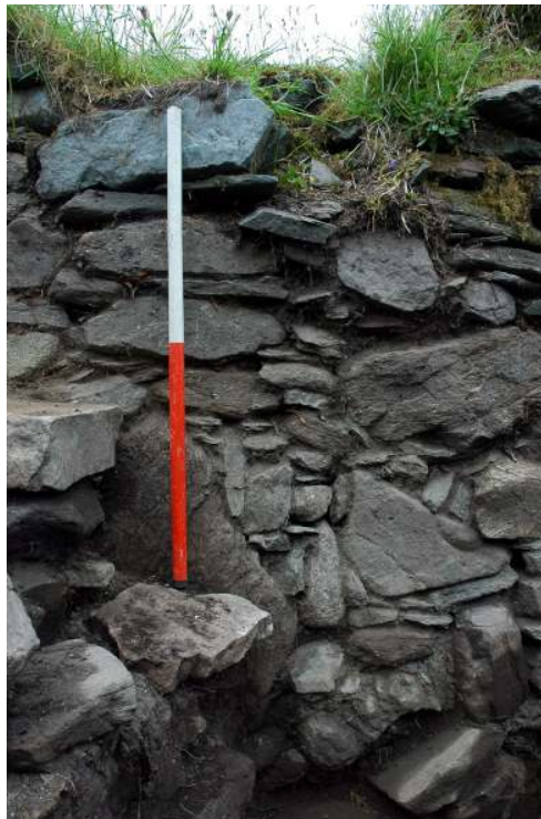
Blocked cruck-slot
