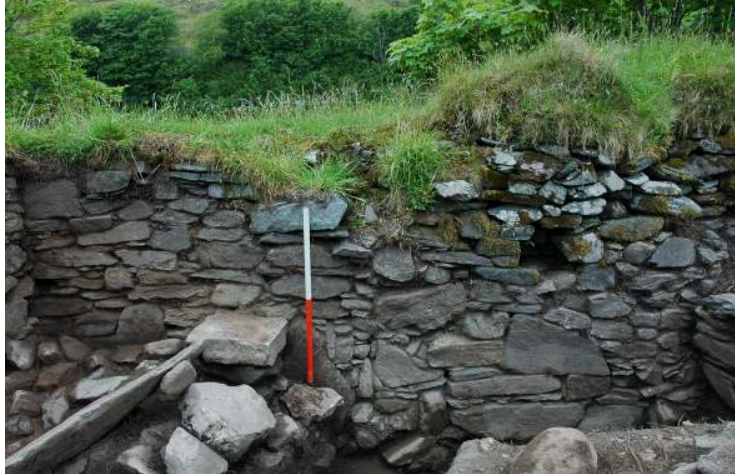
Structure 5 East facing wall
