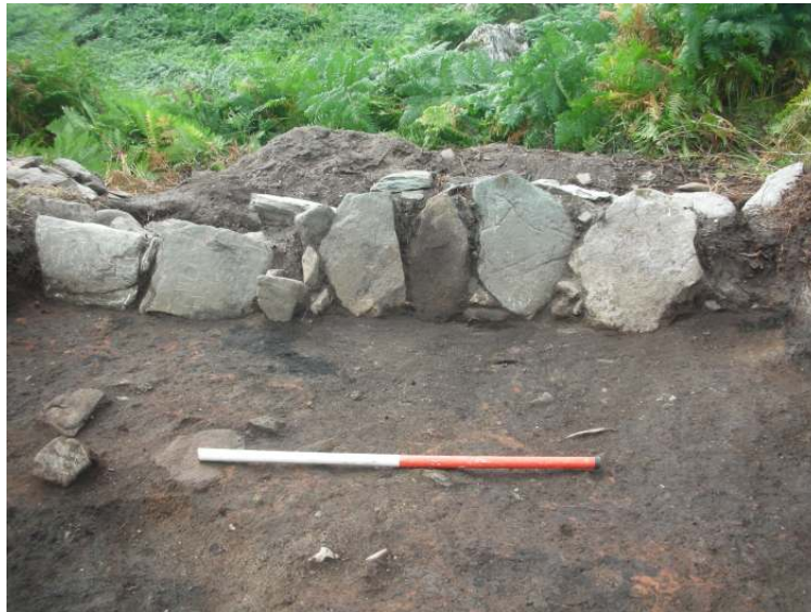
Structure 6, wall rebuild [195]
