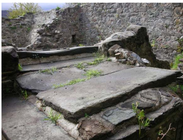
Stair landing at stones-floor level
