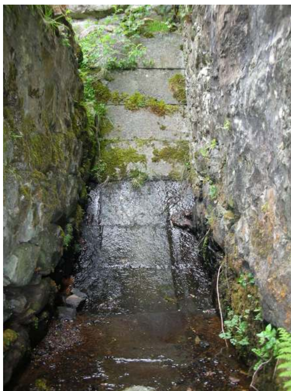
Wheel grooves worn in stone lined lade
