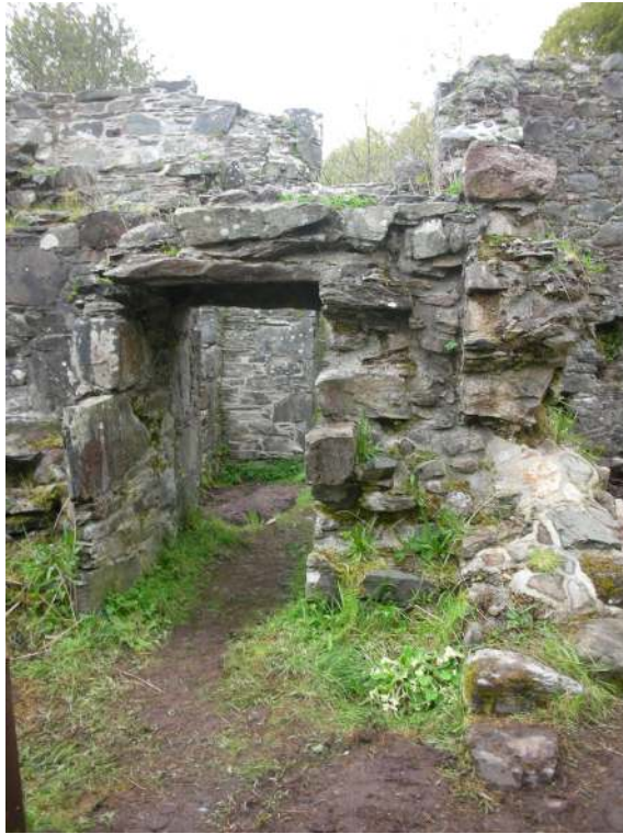
Ground floor door into kiln
