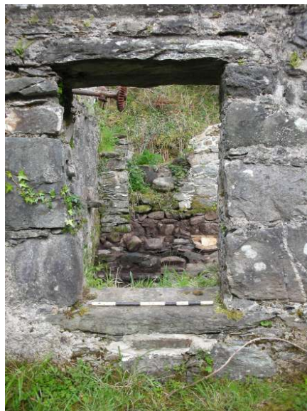
Ground floor window in SE wall
