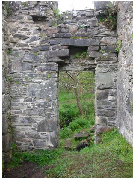
Ground floor door of kiln
