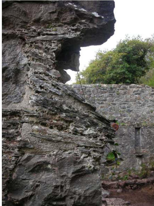
Loading-door arch spring
